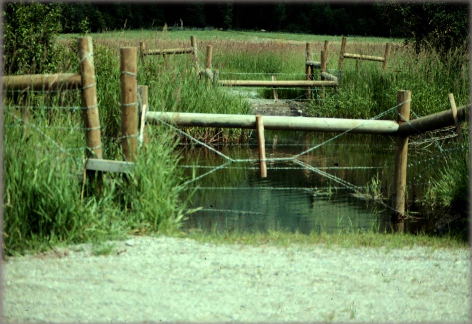
Livestock Access Point Allows Debris Flow and Limits Livestock Access to Stream Channel
