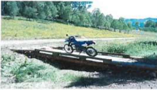
Are the trail structures effective?
