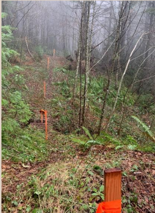
Road P-Line Staked Out & Surveyed
