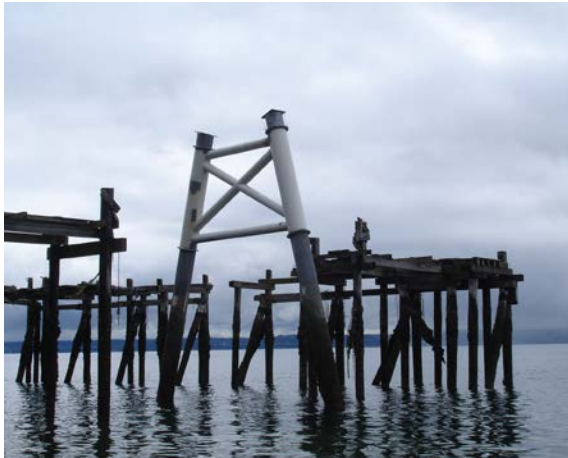
This pile structure was located on the Maury Island shoreline and was removed. Structures such as these altered water flow and sedimentation.
