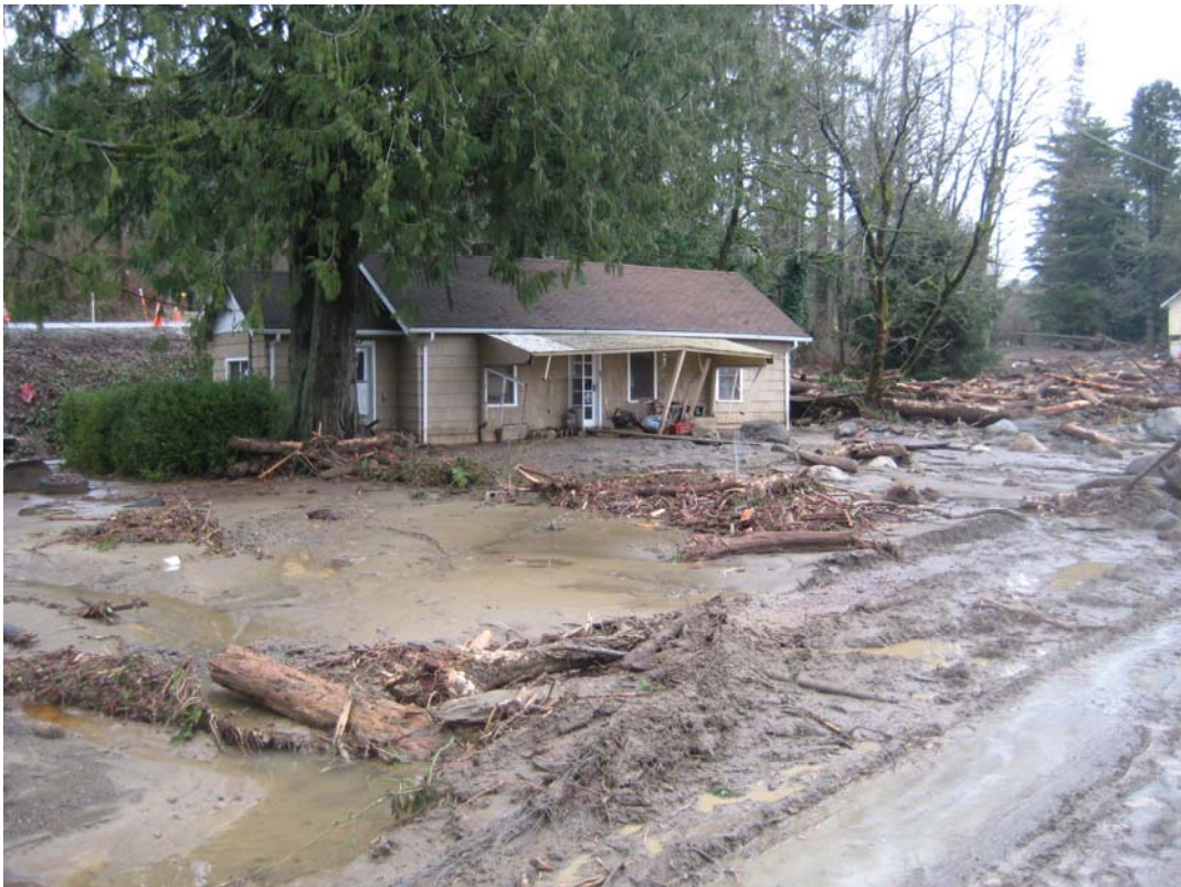
Figure 9. Photograph of Johnson Residence Post Debris Flood. Photograph taken facing northeast.
