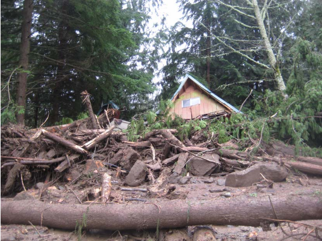
Figure 7. Photograph of Brester Residence Post Debris Flood. Photograph taken facing west.
