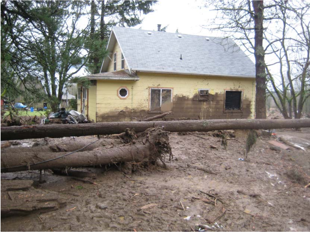
Figure 12. Photograph of Monaghan Residence Post Debris Flood. Photograph taken facing southeast.
