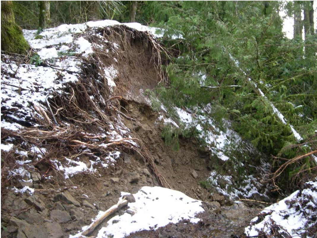
Figure 6. Photograph of Debris Flood Point-of-Initiation, Dam Break Site. Photograph taken facing southeast.
