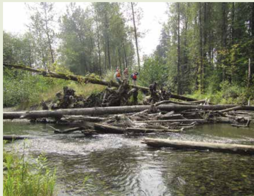
Engineered log jam in the Sultan River. Large woody debris projects like this support healthy riparian ecosystems.
