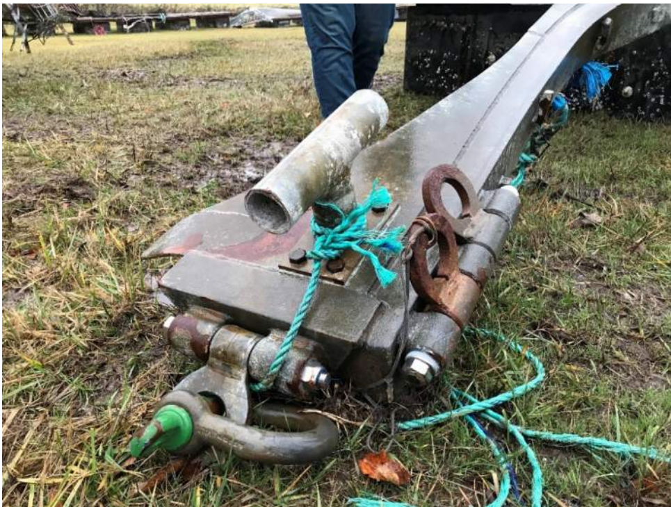
Figure 7.15 –Corner of Outrigger Float – Northeast Corner of pen 225 (Source: DNR) Note intact pad eyes at the mooring brackets.
