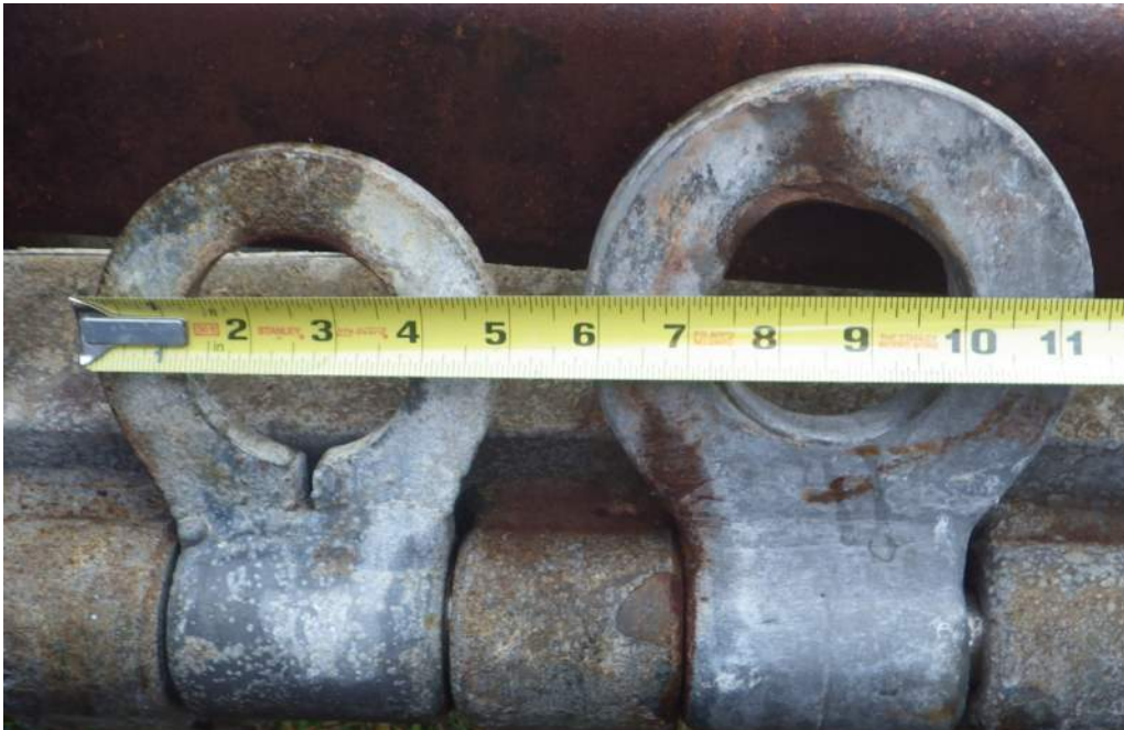
Figure 7.7 – Pad eyes of varying sizes on same mooring bracket (Source: Mott MacDonald)
