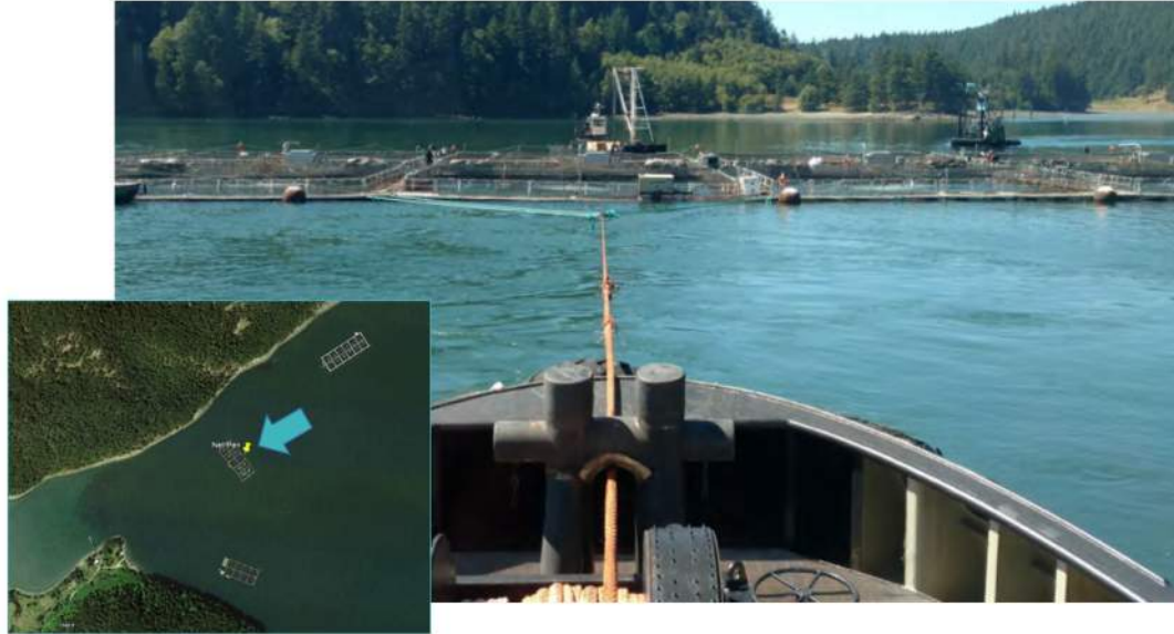
Figure 4.3 – Net Pen #2 being stabilized by Millennium Star (July 2017) (Note reduced freeboard at the floats where the two lines are applying concentrated pulling force.) (Source: Harley Marine and Google Earth)
