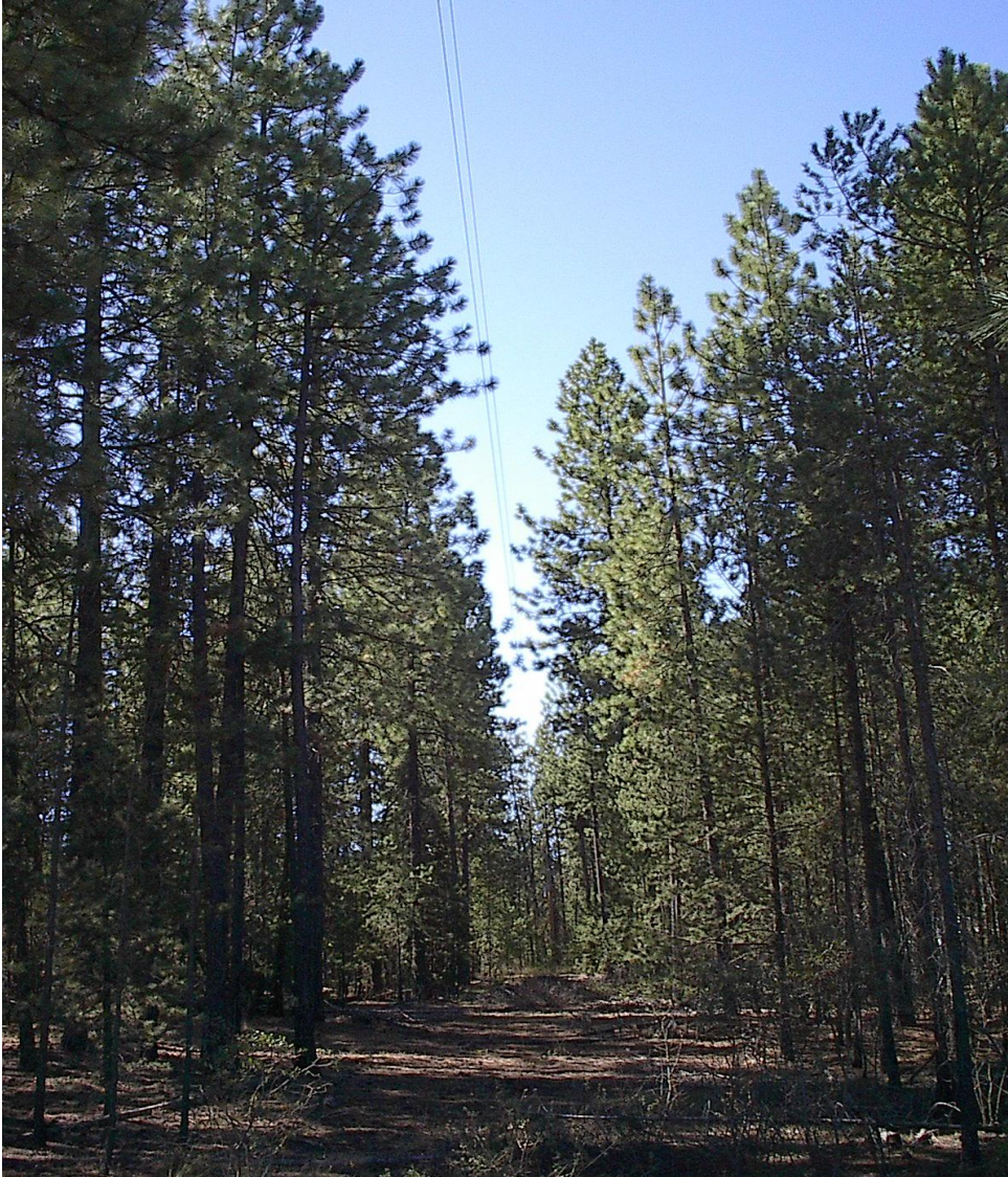
Inadequate example of power line maintenance
