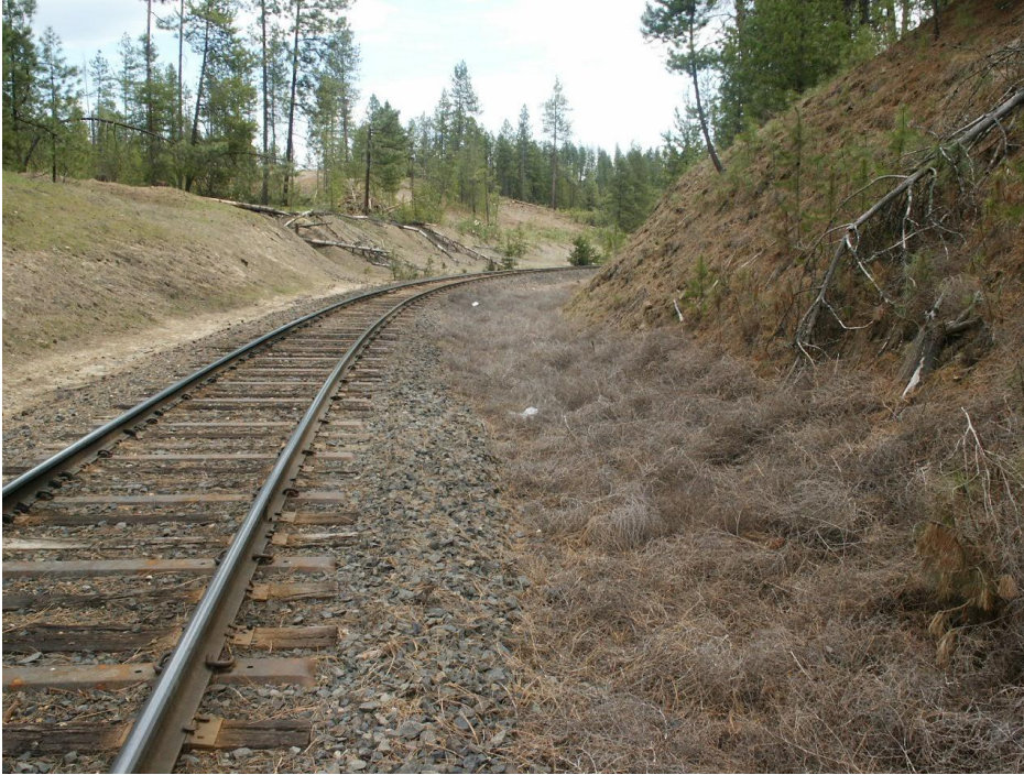
Inadequate railroad right of way clean-up
