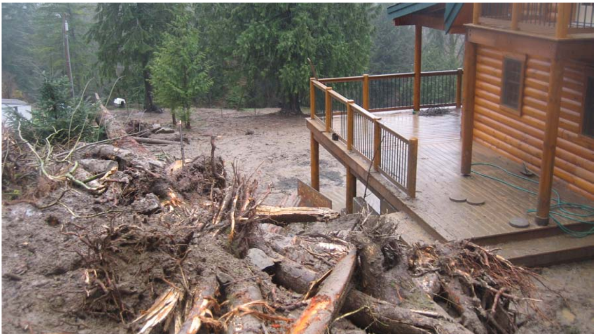
Figure 8. Debris piled near the southeast corner of the home. Note broken ballusters in deck railing. View looking west. (Photo by Doug Hooks, 2009)
