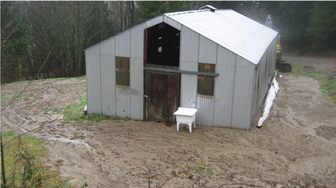
Figure 10. Lower BDS deposition area illustrating flow of debris around out building below the house. View looking northwest. (Photo by Doug Hooks, 2009)
