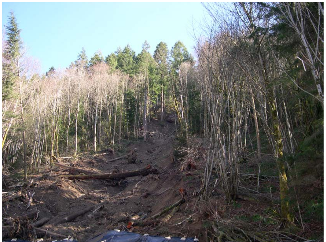
Figure 6. BDS path and upper portion of debris avalanche scar viewed from the bottom of the hill. View facing east. (Photo by John Coyle, 2009)
