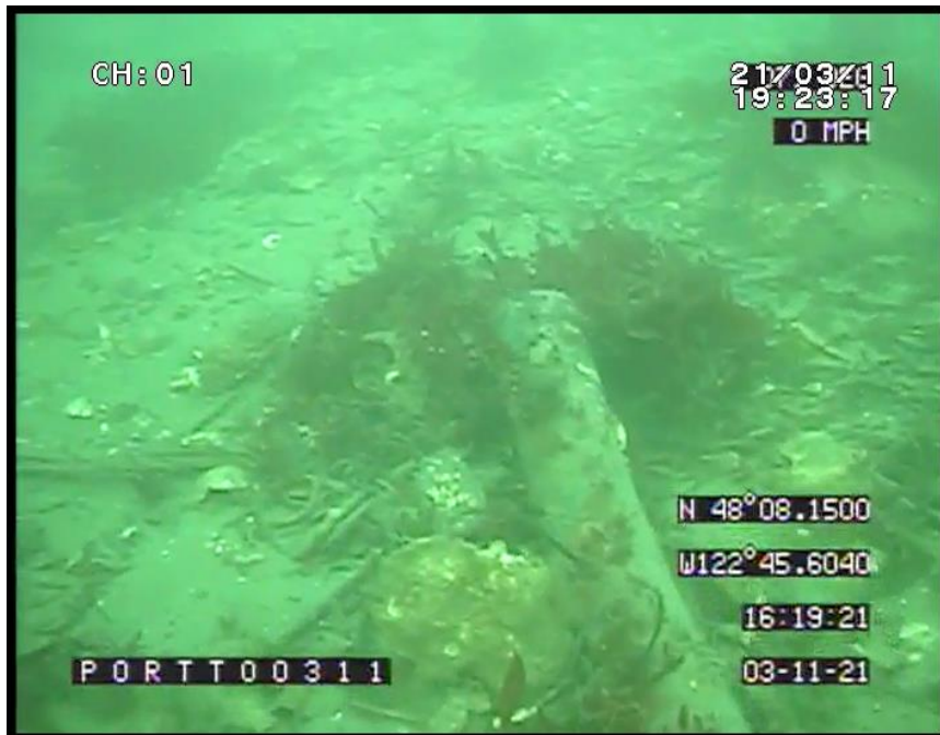
Figure 10. Concrete piling buried in sediment at reef site
