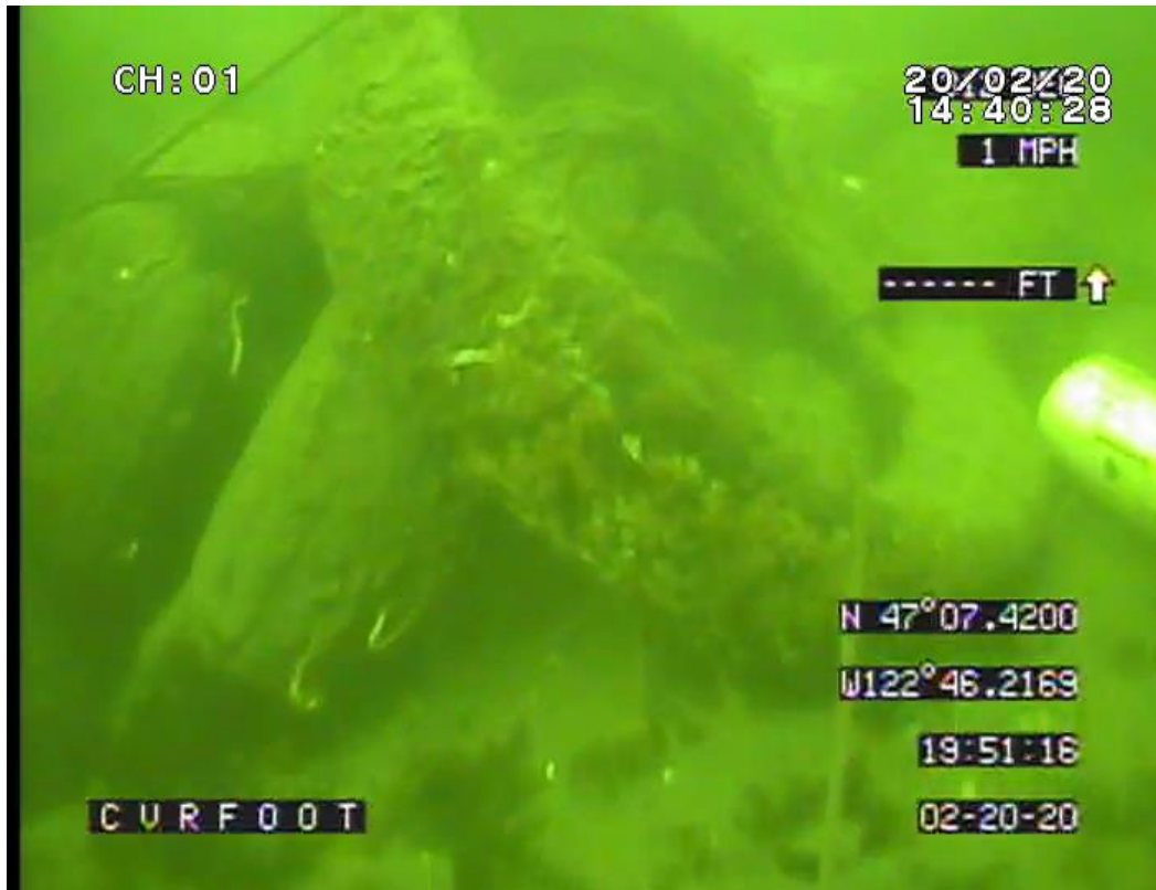
Figure 163. One of many groupings of tires where rope banding has broken, allowing tires to fall apart.
