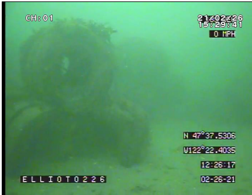
Figure 38. Pyramid - stacked tires present at the Elliott Bay Site. Pyramids are created from 8 - 10 tire barrel rows. Two barrels are connected to a "peak" barrel with polypropylene line. Tires on bottom row appear to be buried up to 1/4 into the sediment.
