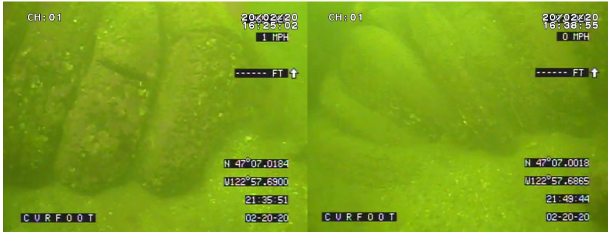
Figure 170. Eld Inlet tire bundles that represent tire bundling, burial levels, and tire degradation typical of the nodes/piles found in the reef.
