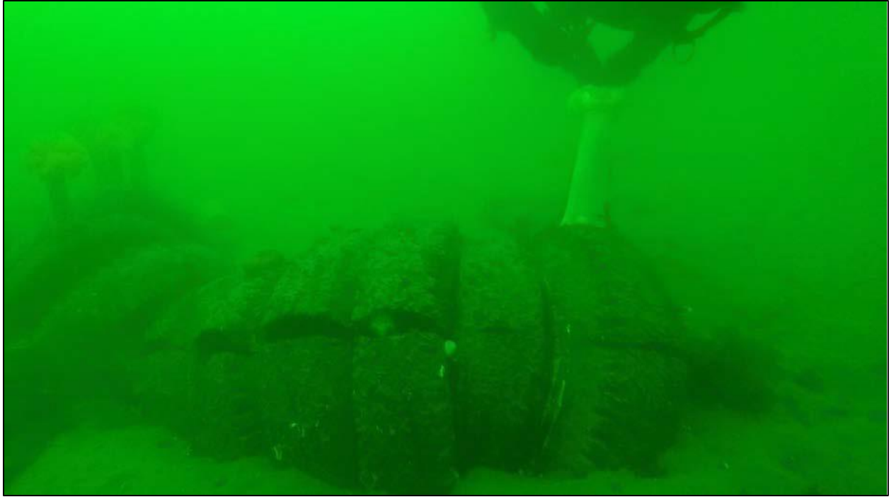
Figure 144. Horizontal bundle of eight tires. Tires appear to have been intentionally slashed on placement. Photo taken by DNR divers.
