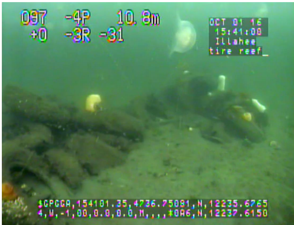
Figure 59. Image from 2016, captured with WDFW ROV. Single layers of tires buried up to 1/2 were present throughout the Illahee reef.
