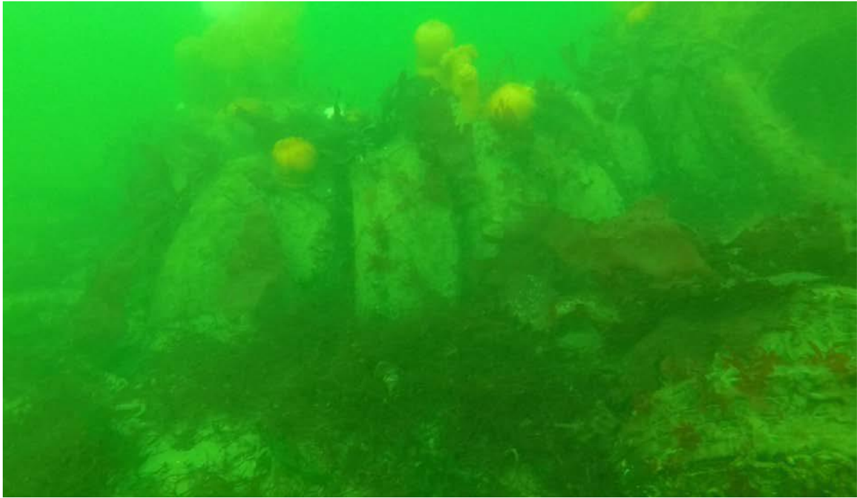
Figure 136. DNR diver survey: barrel-grouped tires that are buried up to 50% in sediment
