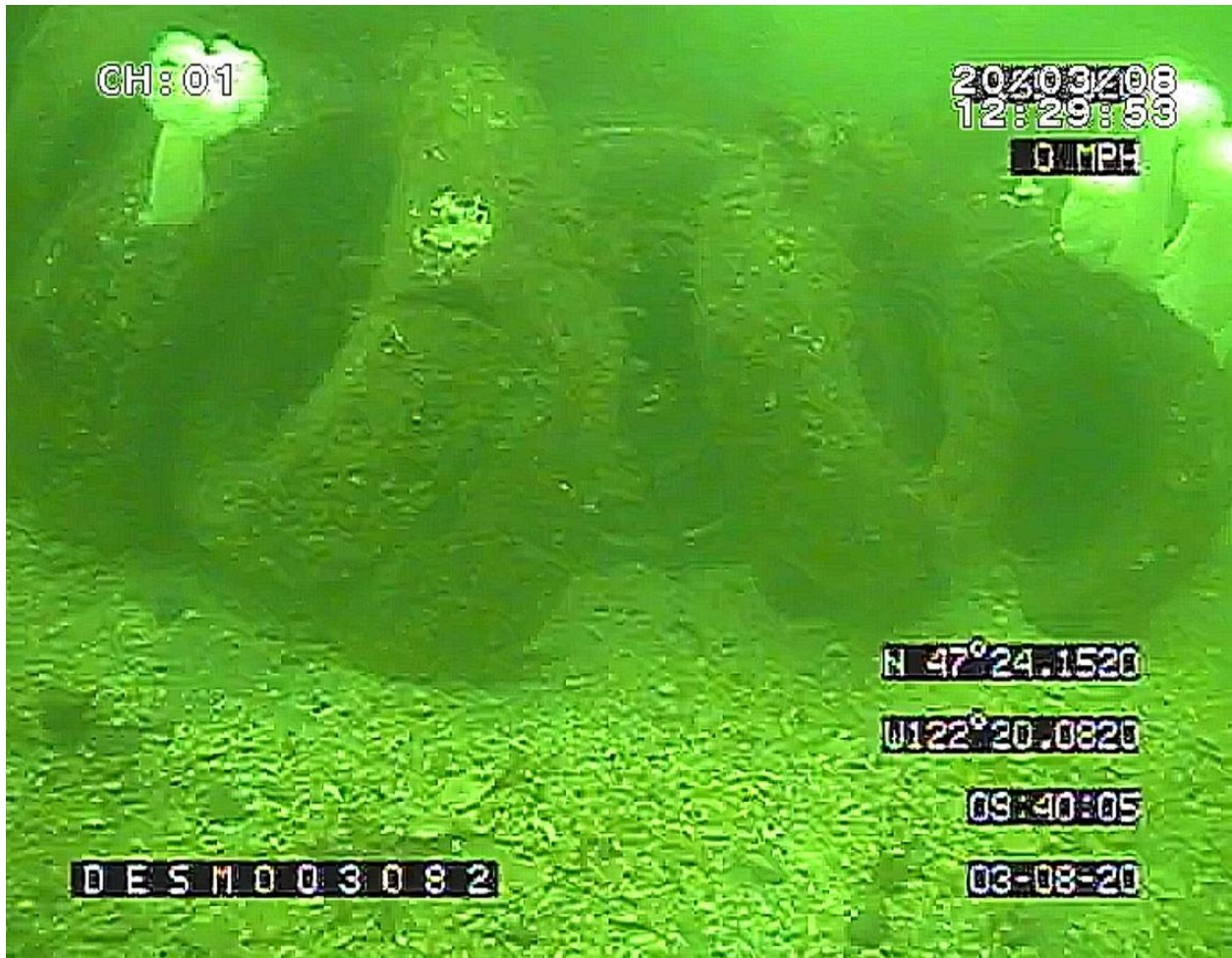
Figure 68. Barrel stacked bundles of tires that have begun to disband and separate from original placement.
