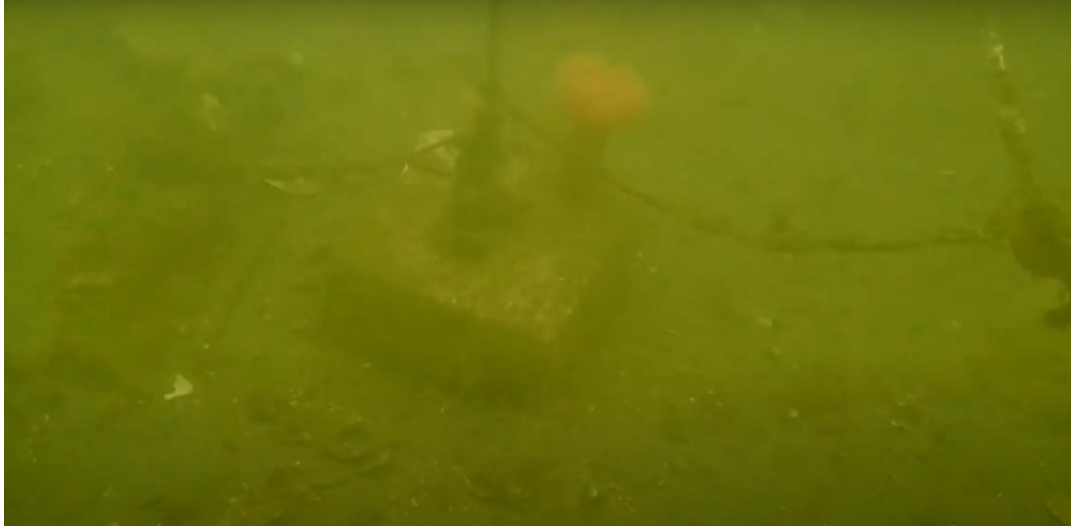
Figure 96. Concrete anchor found in the vicinity of the tire reef. It is unclear whether this was placed to anchor tires, or as part of a buoy system delineating the corners of the engineered reef.
