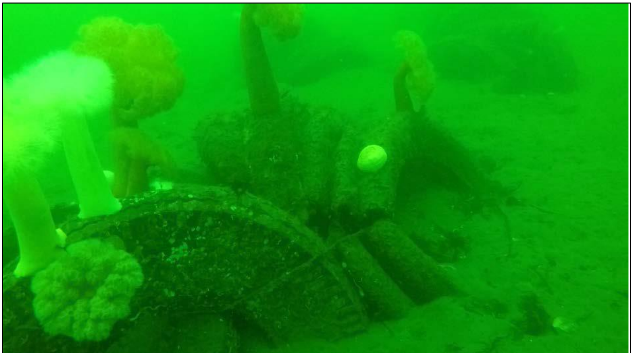
Figure 145. Tolmie Reef tire bundles buried 50%. Bundle in photo is banded with three-strand polypropylene. Photo taken by DNR divers.
