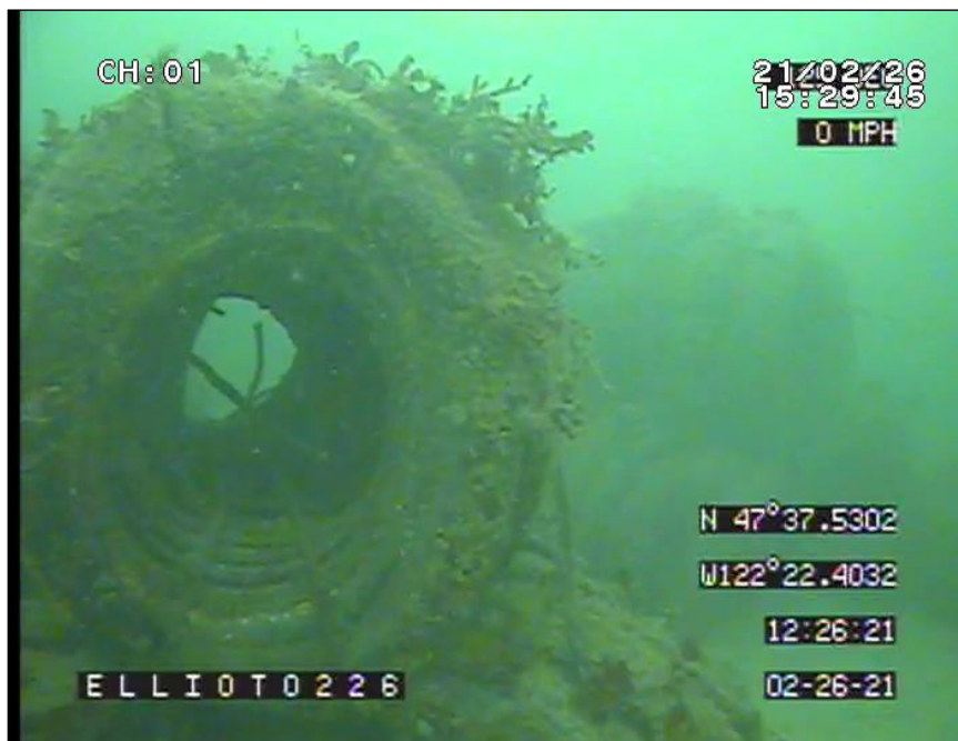
Figure 39. Tires banded in a pyramid formation are banded with multiple sections of polypropylene line.
