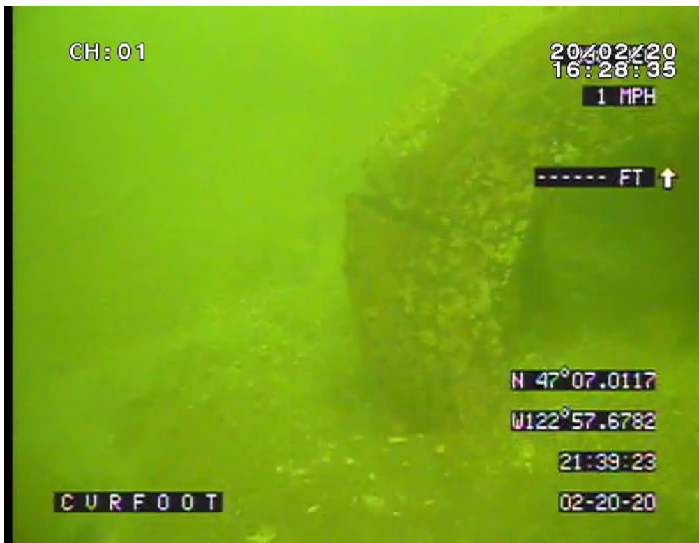
Figure 173. Tires at the Frye Cove reef site are generally in poor condition. This is an example of a tire that is buried ~ 30% in sediment, with slash for air escapement.
