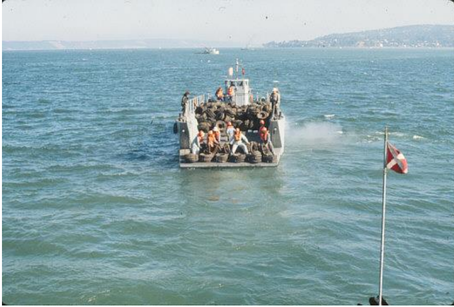
Figure 102. Tires being deployed at the Old Town Dock reef (Date Unknown).
