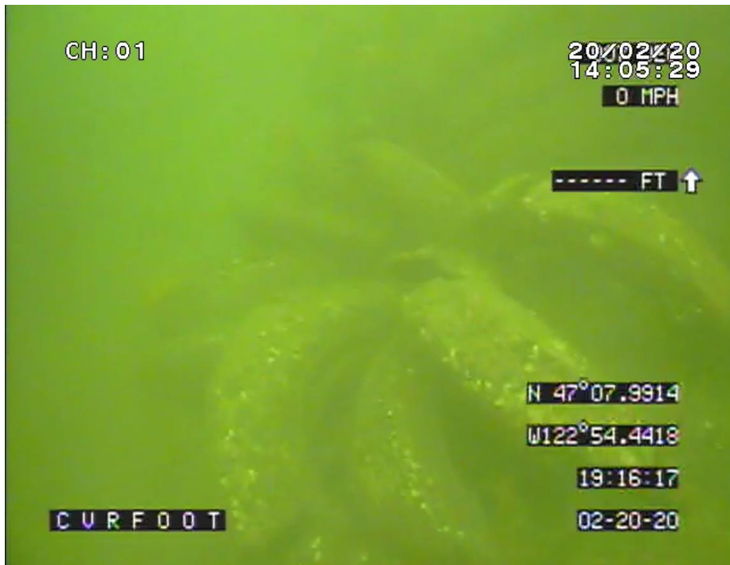
Figure 155. Tires that have broken apart from their bundles.
