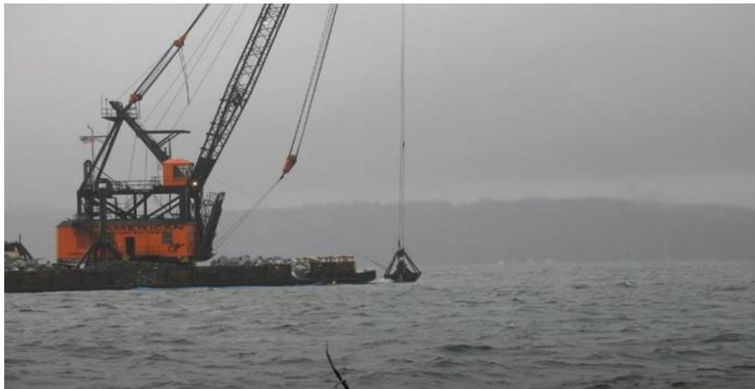
Figure 87. Photo taken from Saltwater State Park in 2006. Boulders and concrete structure were placed in piles to create a well-known diving reef.
