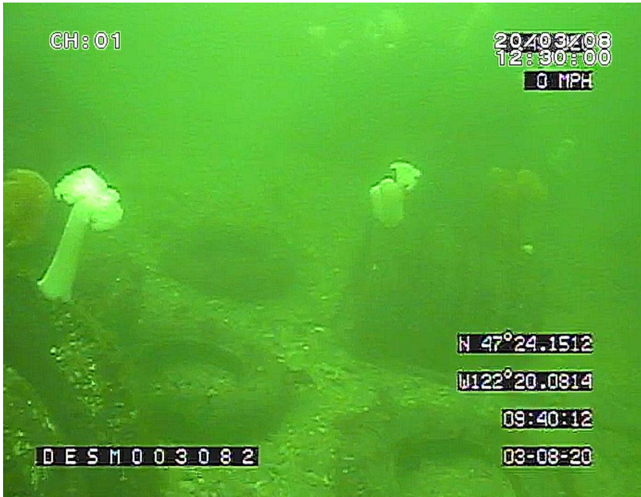
Figure 69. Tires that were likely in a bundle are now separated and lying on the seafloor.
