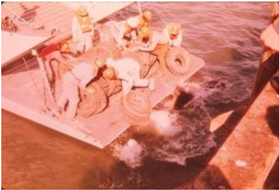
Figure 103. Banded tires being deployed by landing craft at the Old Town Dock reef.
