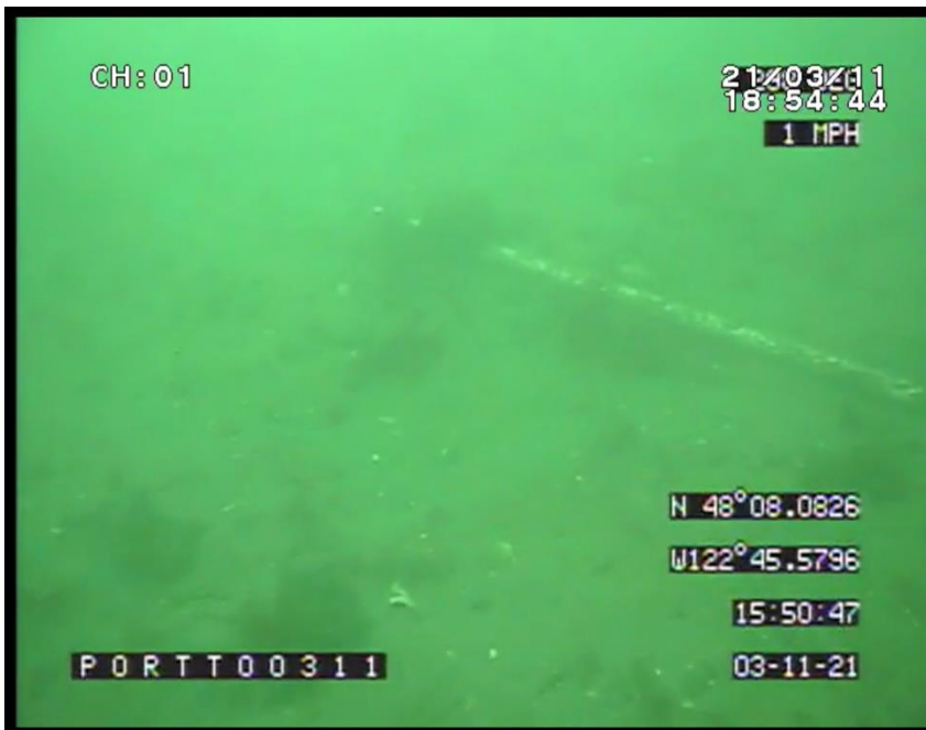
Figure 7. Metal pipe found lying on sediment.
