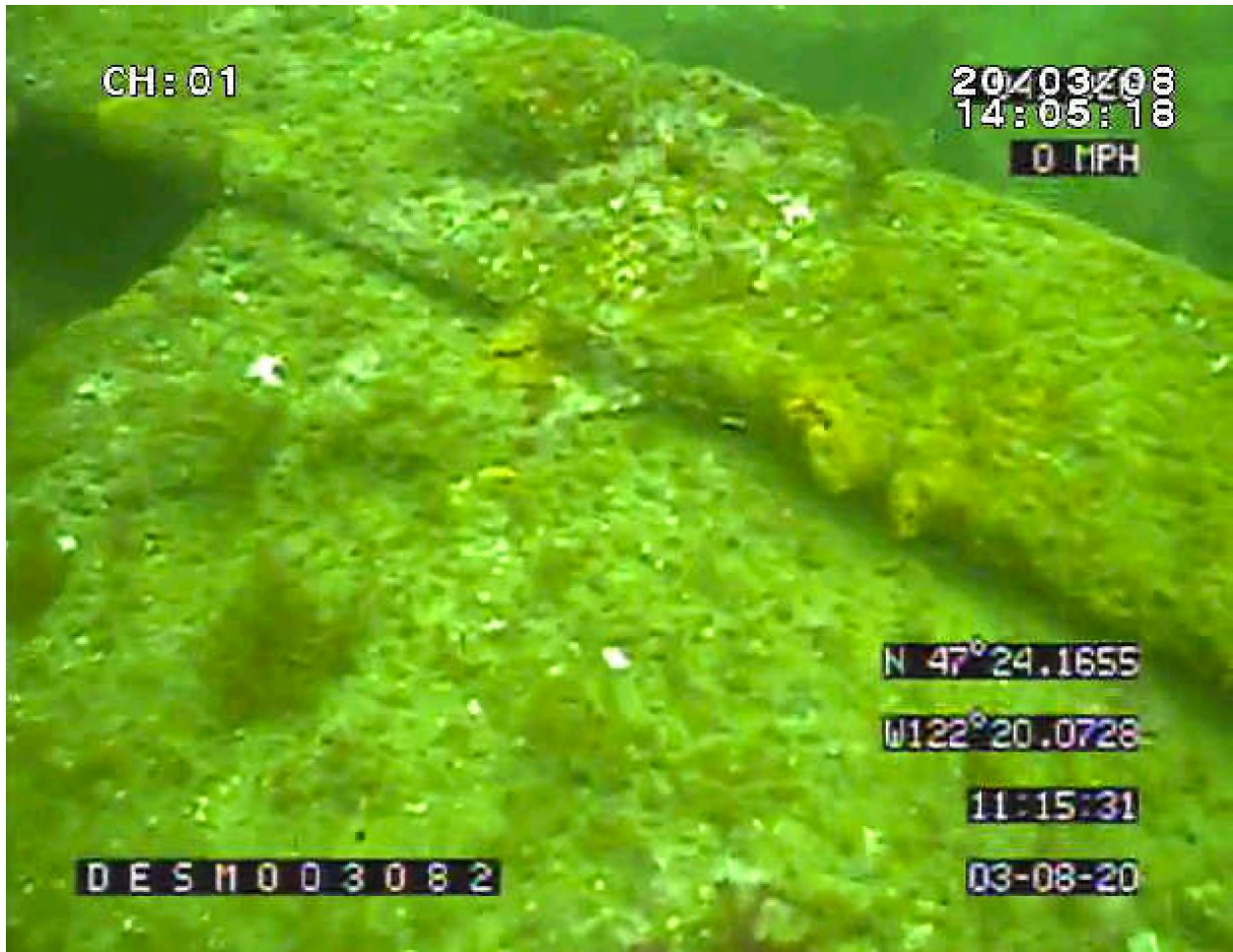
Figure 77. The edge of one of five large concrete or metal dock structures found at the northern portion of the artificial reef (refer to figure 1).
