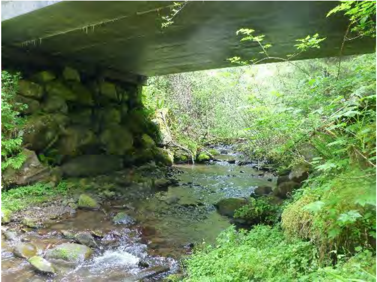
Stream gage station in basin 694 at mid flow.
