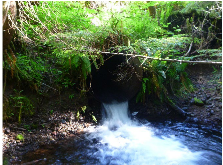
Figure 3. Bear Creek culvert prior to removal.
