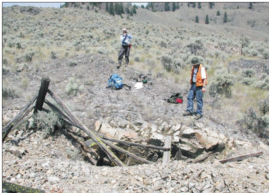
Figure 3. Unnamed open mine shaft approximately 50 feet deep on Palmer Mountain in Okanogan County. Open shafts such as this can be extremely hazardous because of loose material around the collar, rotting timbers, and vertical depths that could be fatal in a fall.
