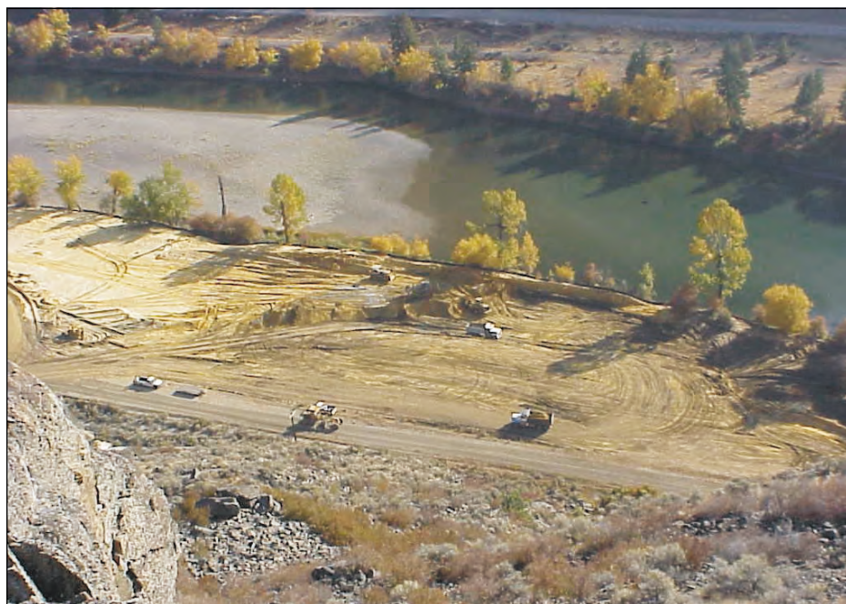
Figure 4. Tailings deposited along the banks of the Similkameen River from the Kaaba Texas mine were removed and the banks revegetated in 1999 and 2000. The revegetation was the result of an interagency cooperation between BLM, EPA, DOE, and DNR. The metal-bearing tailings were loaded onto trucks and hauled to an upland repository where metals would not be released to the environment. Approximately 80,000 cubic yards of tailings were removed. (Photo courtesy of EPA Region X.)
