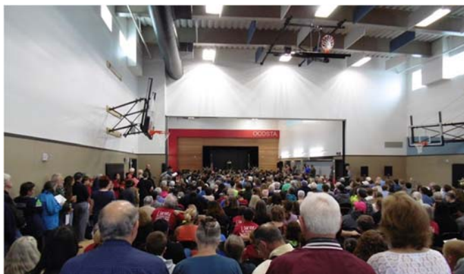
A full house of close to 500 attended the Ocosta Elementary School dedication. The rooftop of this combined gym and cafeteria building is the tsunami vertical evacuation refuge. Credit: Ted Buehner
