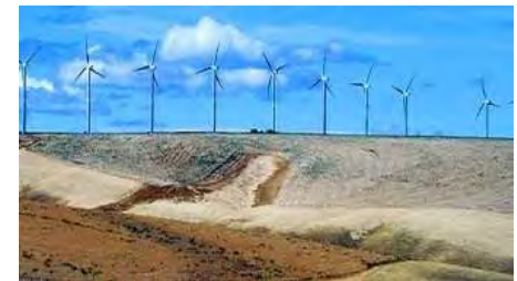
IMAGE SHOWS WIND TURBINES ON STATE-TRUST LANDS FOR PRODUCING ENERGY. SOURCE: WA STATE DNR
