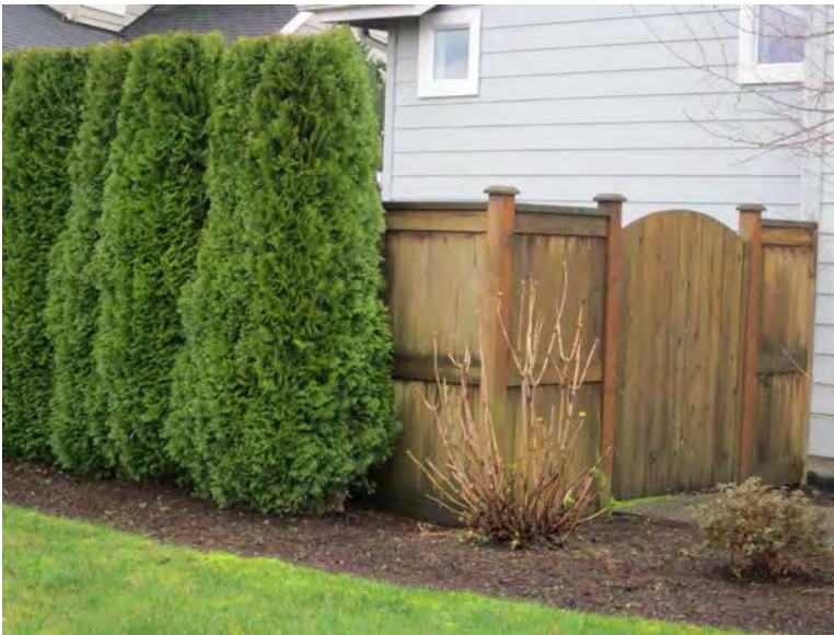
Figure 5-16: Wooden fences connected to structures can spread fire.
