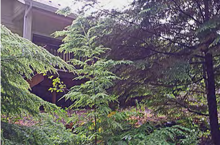
Figures 5-15: Raised wooden decks can accumulate flammable material underneath.
