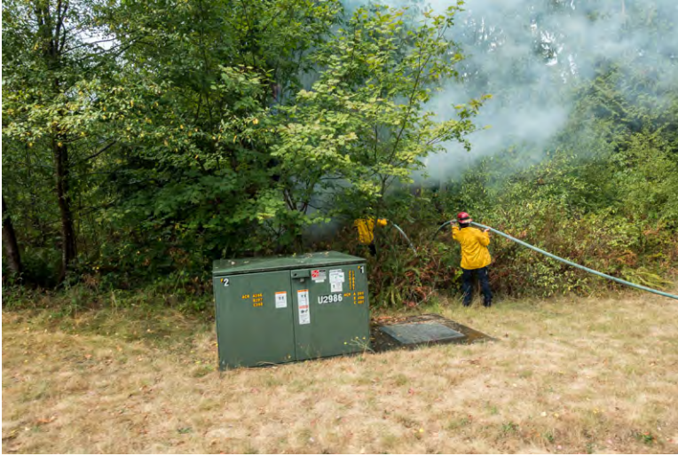
Figure 5-2: Fire crew extinguishing tree fire following lightning strike in August, 2015
