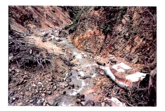
This culvert in Milky Creek was obviously inadequate to handle the water, sediment, and debris load transported down the channel.
