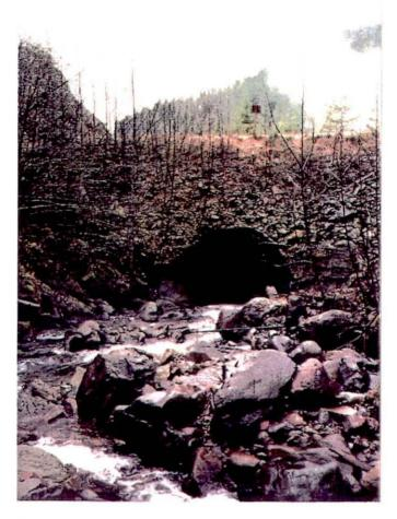
This culvert on East Fork Silver Creek probably has adequate capacity to handle peak flows. The rust line, visible on the left side of the culvert, is well below one-quarter the height of the culvert and there is no indication of erosion around the culvert inlet.
