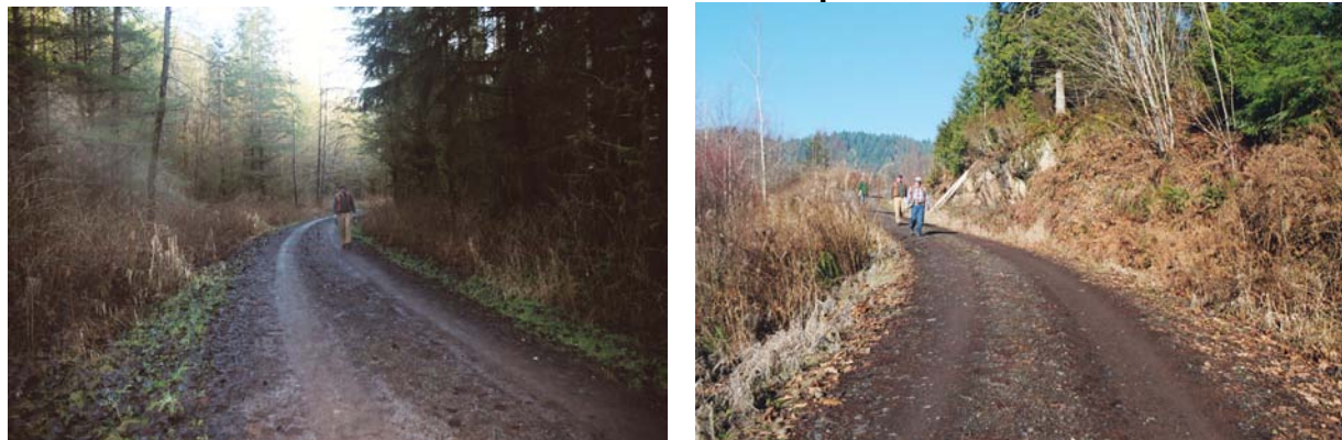
Plate D-2. Stossel Creek spur road.
