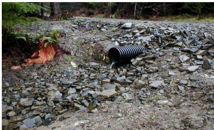
Figure C-7. Rip Rap Protection at Culvert Outfall
