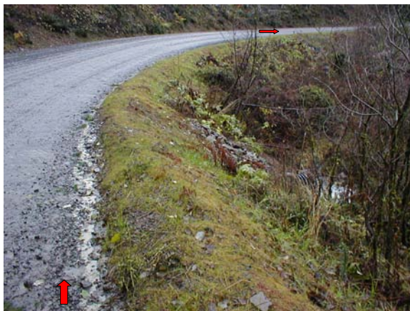
Figure C-6. Berm on Outside Shoulder of Road
