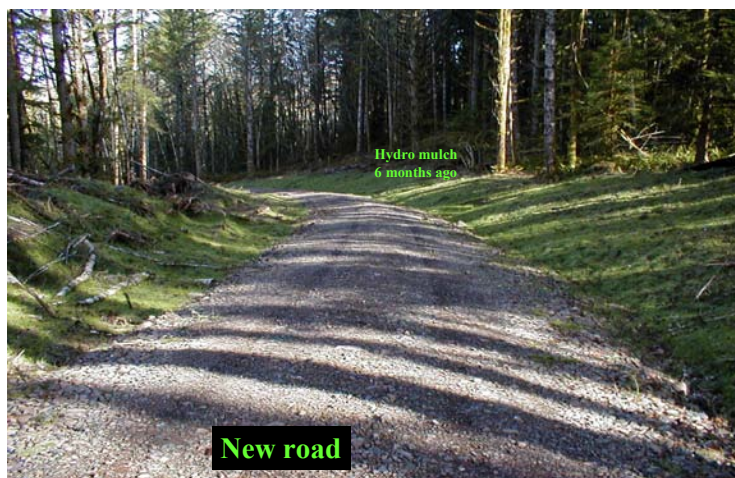
Figure C-3. Hydromulched Cutslopes
