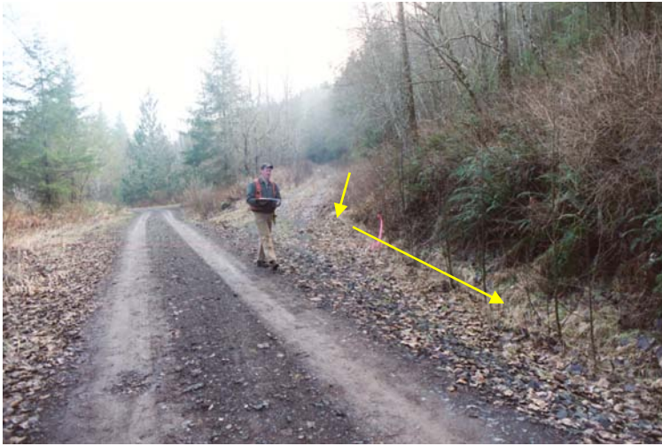
Figure 5. Example of a road segment draining to another segment.
