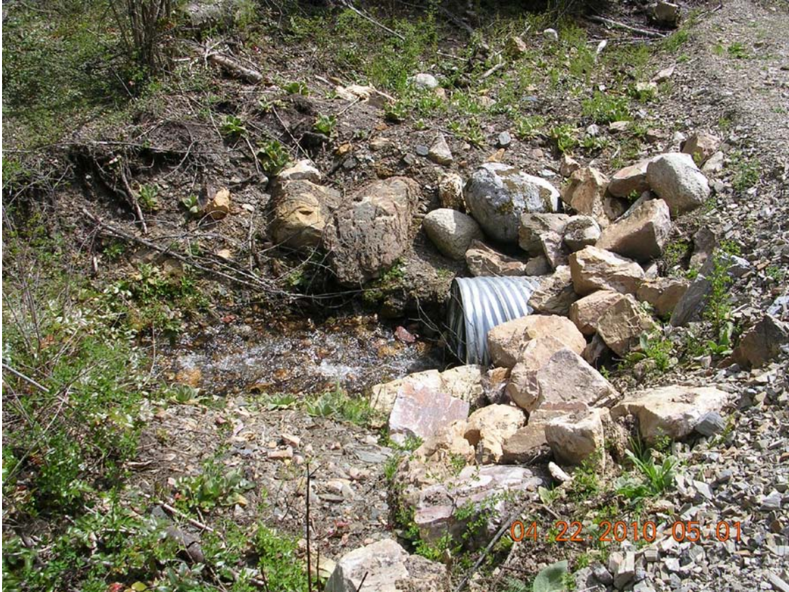
Well protected type Np stream crossing in new road construction.
