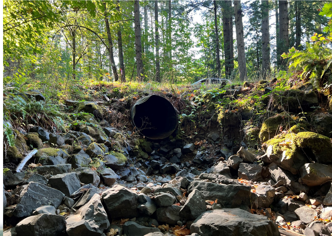
Downstream of FPB tour site
