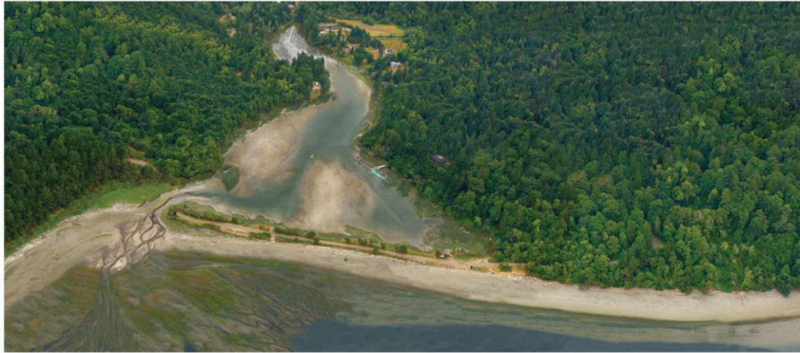
Post construction (low tide)
