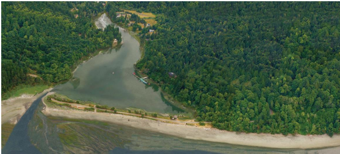
Post construction (High tide)
