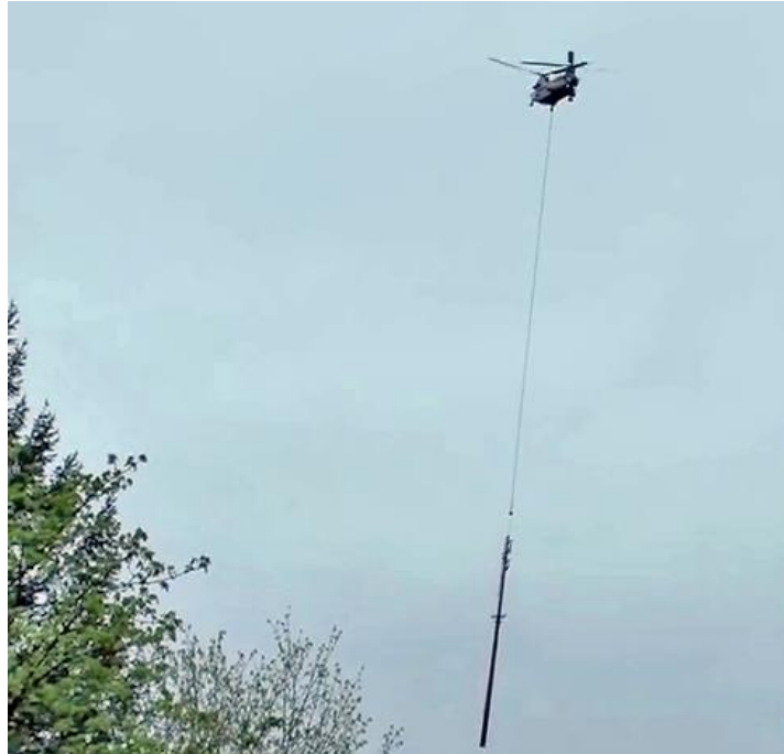
Chinook helicopter transports a replacement structure to a remote portion of transmission line. Photo: BPA
