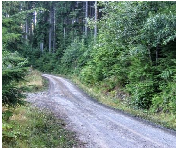
Standard best management practices to minimize erosion include placing crushed surface rock on roads. Photo: DNR
