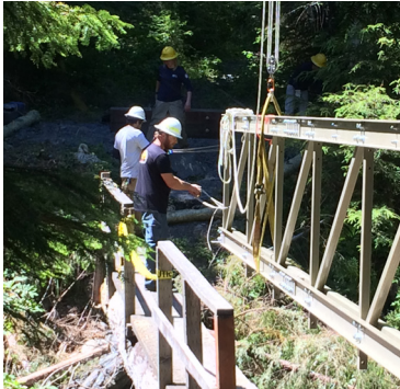
Top: Gothic Basin Trail sign; Bottom: Ashland Lakes bridge installation (2015).
