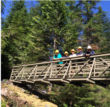
Bottom: New bridge on Ashland Lakes Trail (installed 2015); Top: Sheep Gap Mountain
